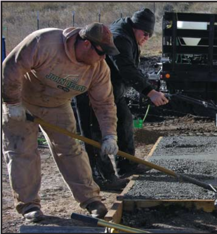
The O&M crew doing concrete work at Arrowwood.
