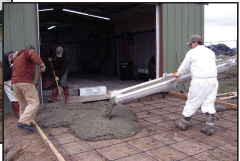
The O&M crew doing concrete work at the McClusky shop.
