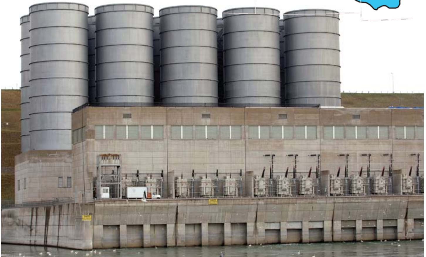
The Garrison Dam power house provides hydropower, one of the original purposes of the 1944 Flood Control Act.
